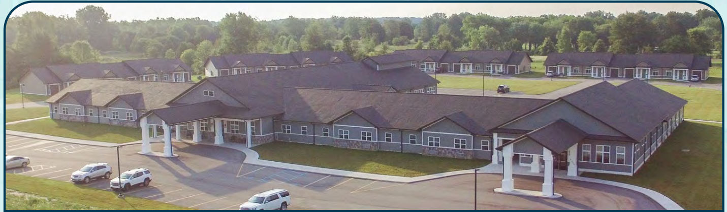
#1 Senior Living Community & #2 Assisted Living Facility The Heartlands
