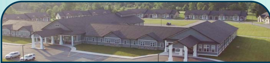
#1 Senior Living Community & #2 Assisted Living Facility The Heartlands
